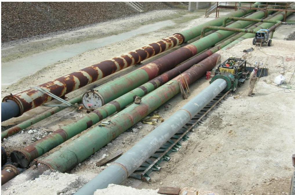
4- 120' bores planned to replace existing casing
