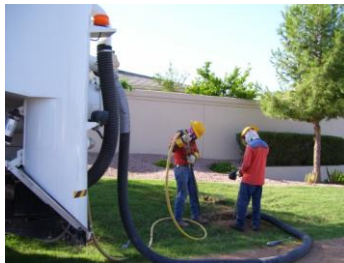
(Vacuum crew exposing utility)
