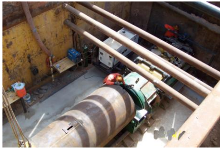
(BMTA & Bore Machine in bore pit)
