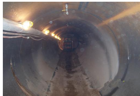
(View looking into tunnel with vent line and lighting)
