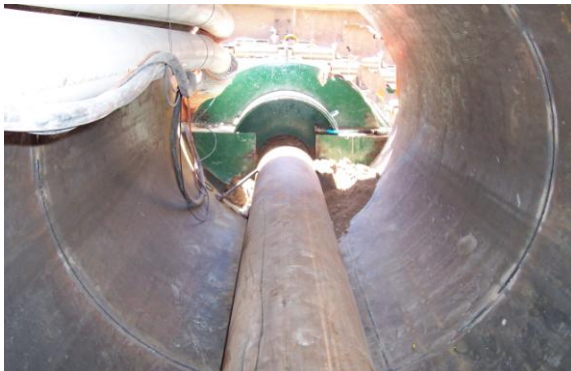
(16" auger/casing used to extract spoils)
