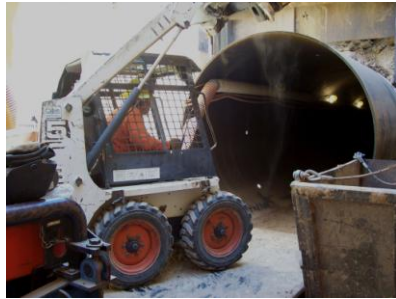
(Skid Steer pumping into spoils bucket)
