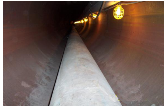
(View inside 500' tunnel)
