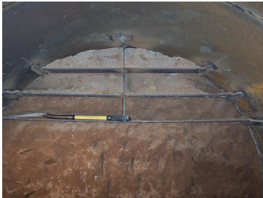
(Tunnel shelf used to control sluffing / cave-in)
