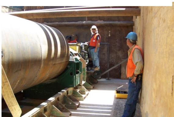
(View of bore pit, track, and bore machine)
