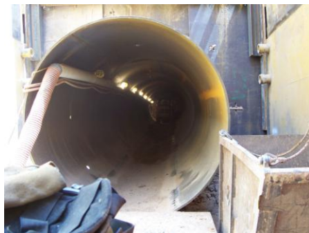
(Landing used for skid steer & pushing casings)
