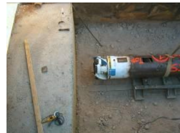
Figure 6: SBU attached to casing.
