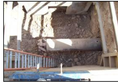
Figure 7: SBU 50' bore pit, 24-in casing
