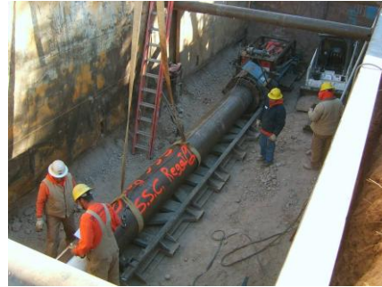
Figure 5 : SBU to install casing for fiber optic
