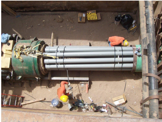
Figure 6: Conduit bundles being pushed into 42" (106.7 cm) casing
