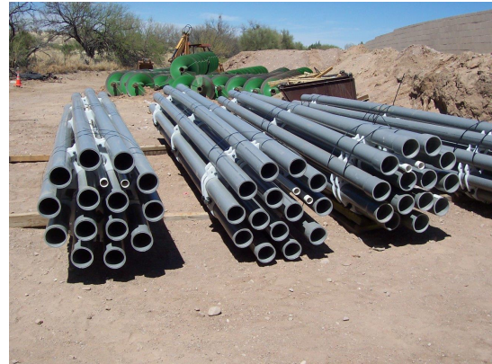
Figure 7: Conduit bundles of 14 – 6" (15.2 cm) Sch 80 PVC
