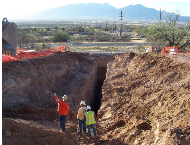
Figure 5: Reception side of crossing, showing 80' (24.5 m) of open cut.
